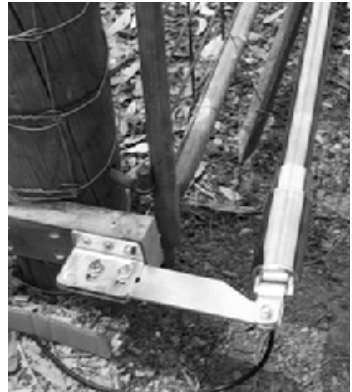
Option A Rear post mounting
