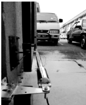
Option B Inside face mounting
